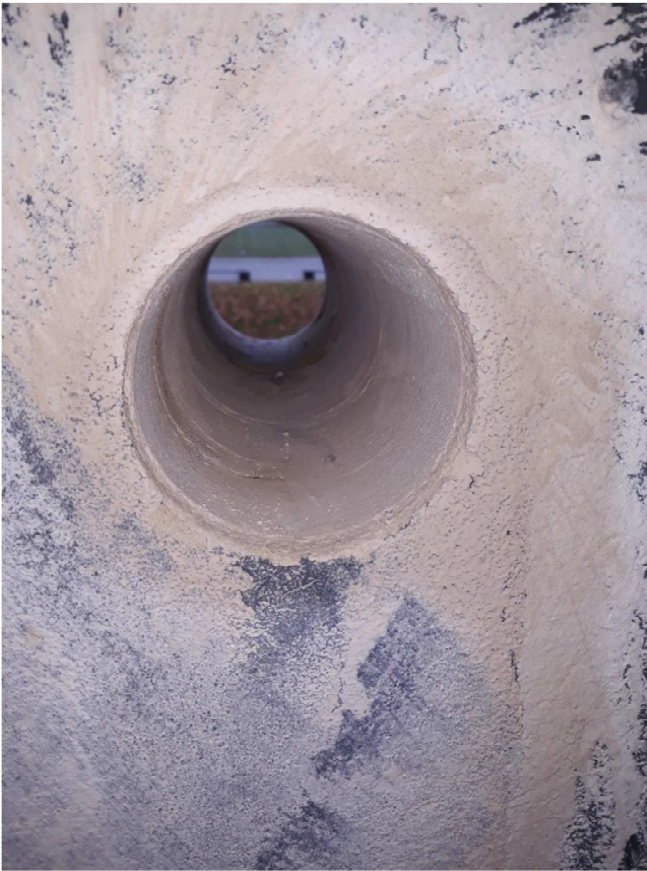
Bohrloch Wand West
